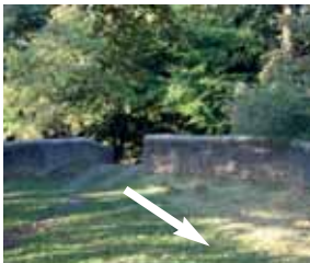
At Bishop Trevors Bridge pause to enjoy the view and gather your strength ...
